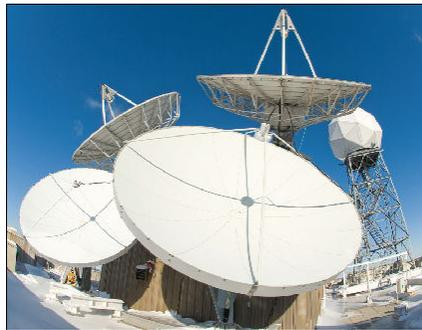
**Figure 2.6.1:** The GOES-10 tracking antenna (center foreground) which sits on top of the SSEC building, amidst the other (fixed) GOES antennas and the MODIS (MODerate Resolution Imaging Spectroradiometer) Direct Broadcast antenna (right).
