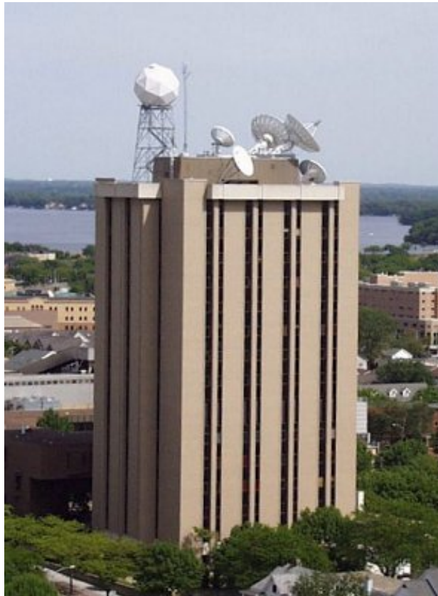
Figure 1: Atmospheric, Oceanic, and Space Science Building which houses SSEC and CIMSS.
