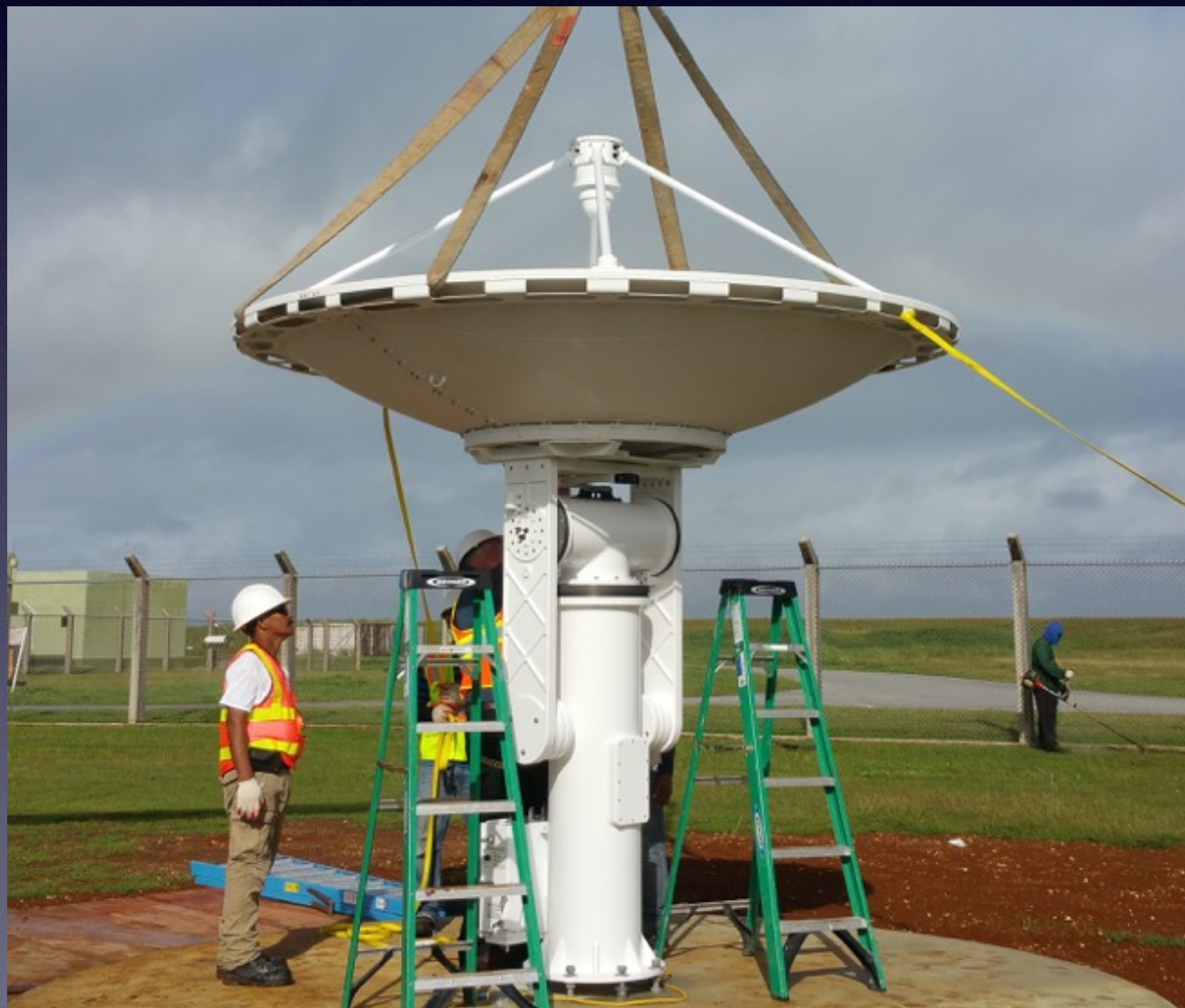
3.0 meter X/L-band Antenna at NWS Guam
