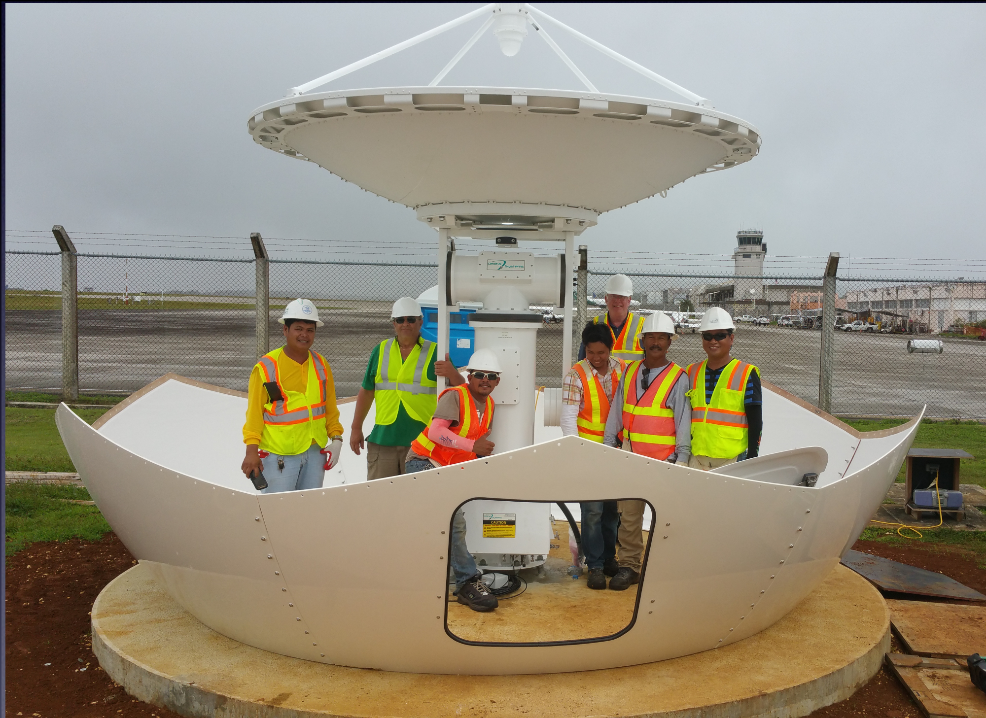
Orbital Systems 3.0-meter X/L-band antenna and positioner NWS Forecast Office Guam
